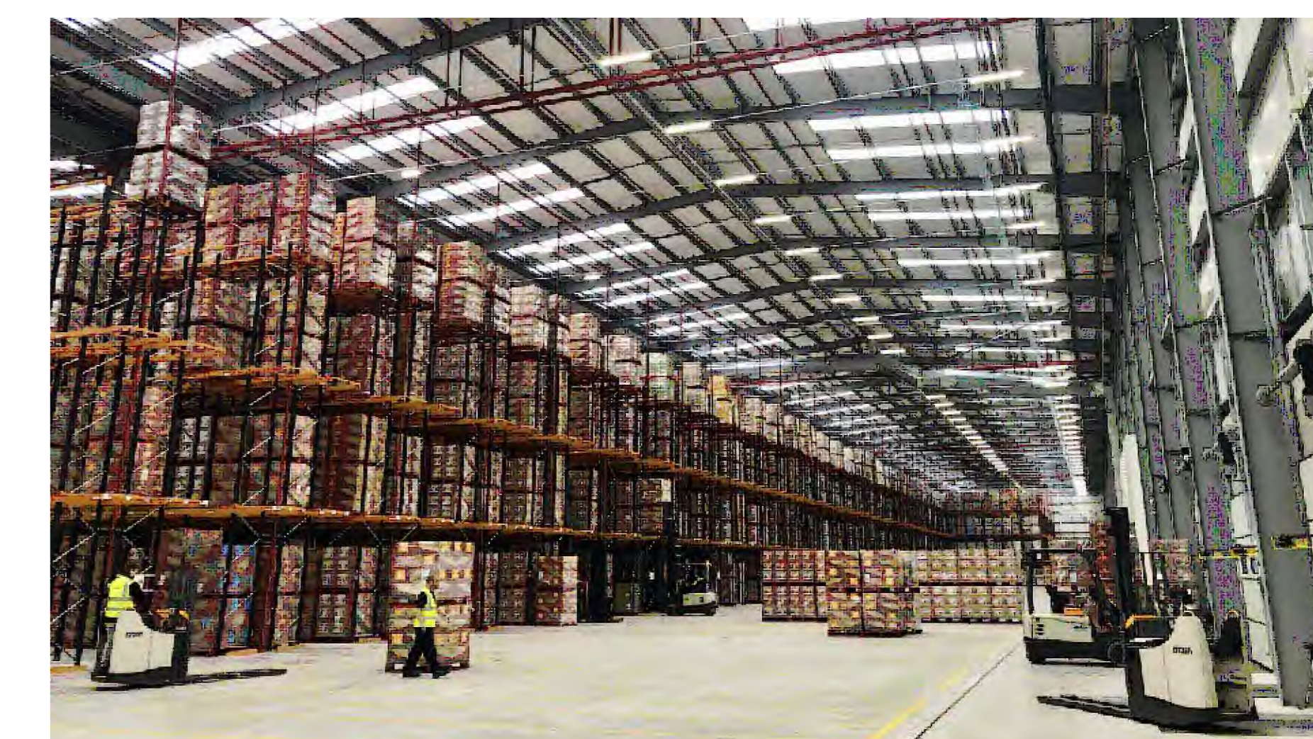
Image 3 - Ground mounted racking system
